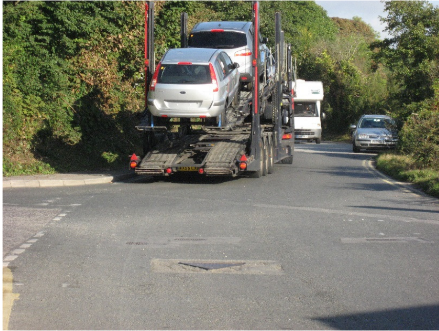
Figure 1 Traffic conflict at the Lighterage Hill/Newham Road junction. Position of parked vehicle contributing to the conflict. (Photograph supplied by the Newham BID committee).
