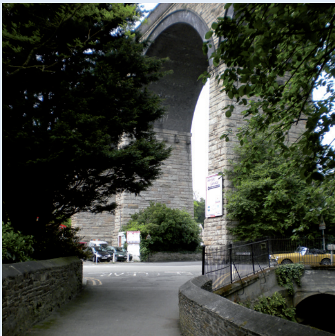
Viaduct before skateboard park
